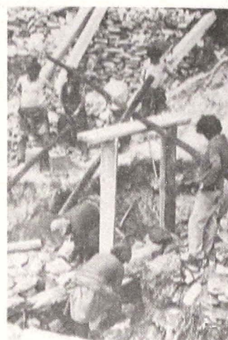
Fig. 32 — Laying of the bastaings
