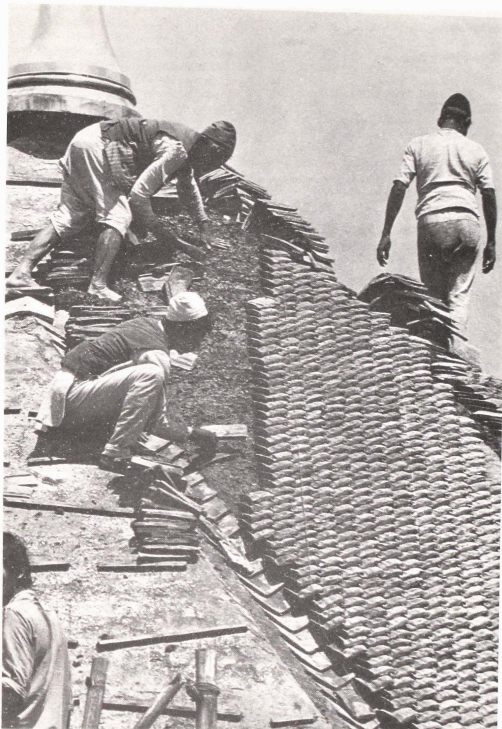
Fig. 34 — Laying of traditional tiles on a temple roof (Cl. J. Sanday)
