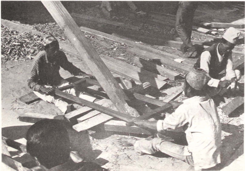
↓ Fig. 33 — Construction of a window (Cl. J. Sanday)
