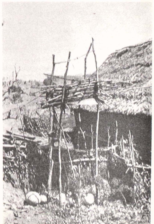
Fig. 7 — Cage on stilts to store Indian potatoes and pumpkins (Cl. M. Gaborieau)
