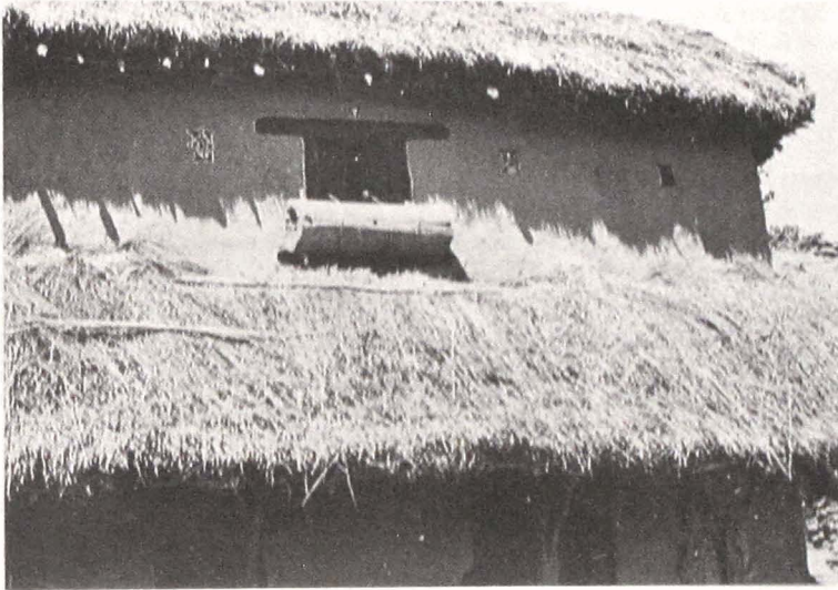
↑ Fig. 14 — Facade wall and opening (Cl. M. Gaborieau)
