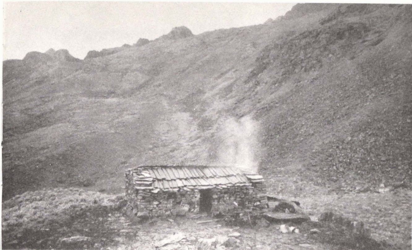
↑ Fig. 1 — Fixed shelter (stone walls) (Cl. P. Alirol)
